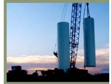
Windmill tower being erected at Bluegrass Ridge in Gentry County, Missouri
